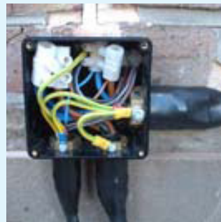
Gland to plastic box connection
