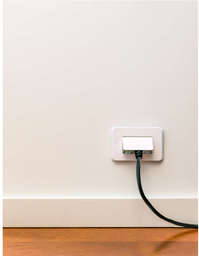
Aesthetically appealing cable management
