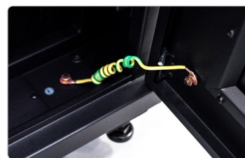
Earth straps on front and rear doors
