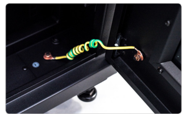
Earth straps on front and rear doors
