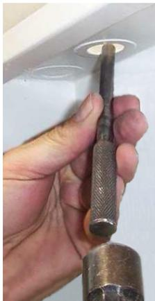
Use a punch or screwdriver and a hammer to remove a knockout
