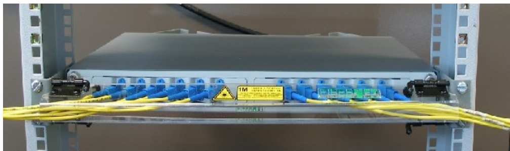
Figure 18. Perspex security front cover for patchcord routing
