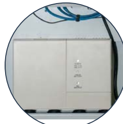
Power supply unit mounting position for NBN battery backup power supply.
