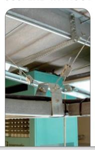
The range consists of a range of wire reels and clips with a choice of Safe Working Load:
