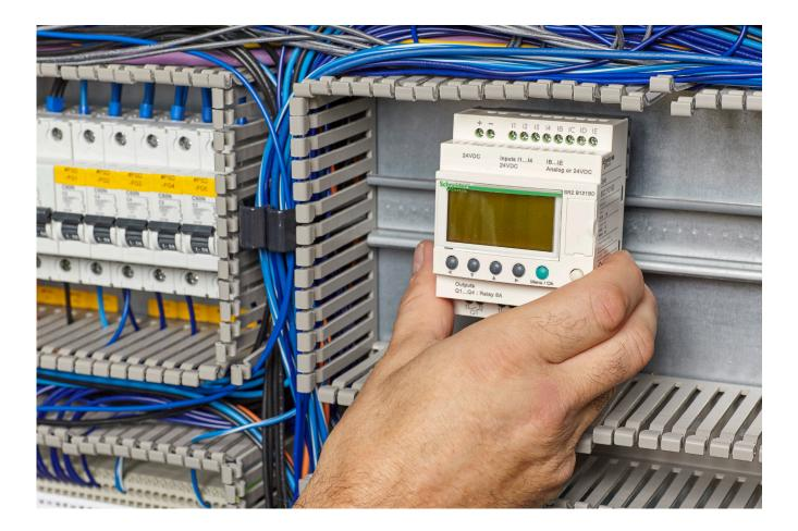
Designed for the management of simple automation systems, Zelio Logic smart relays, with their unique combination of value for money and ease of use, provide a real alternative to solutions based on hard-wired logic or dedicated cards.
