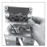
Screw the Clipsal C2000 Series Outlet with the screws supplied in the FPSS packaged box.
