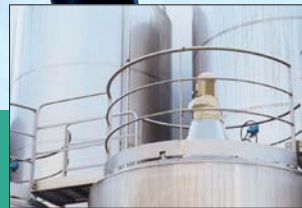
Power supply to motors and pumps
