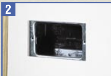
2 After Wall is Mounted, Cut Out Accessory Hole
