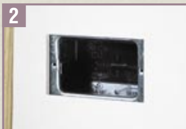
After Wall is Mounted, Cut Out Accessory Hole
