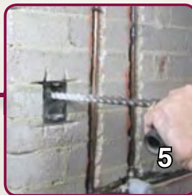
5. Drill hole for cable.
