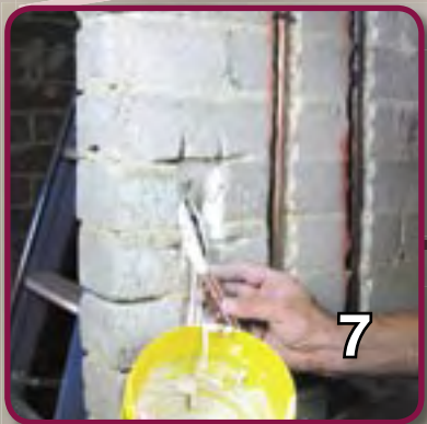
7. Remove wallbox and apply wall/wallbox adhesive.
