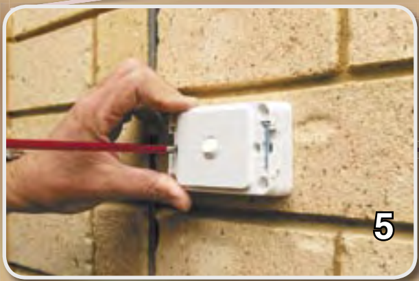
5. Screw fix product to 2449ASD Spacer Block.
