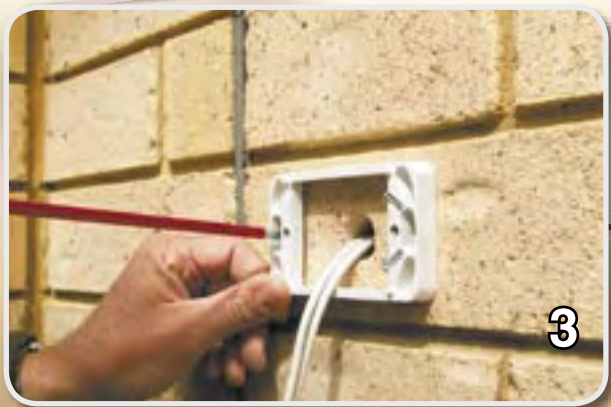
3. Screw fix 2449ASD Spacer Block.
