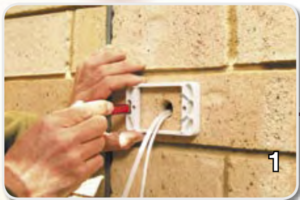
1. Mark out mounting position.
