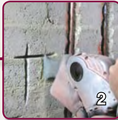
2. Cut or drill out along wall markings.
