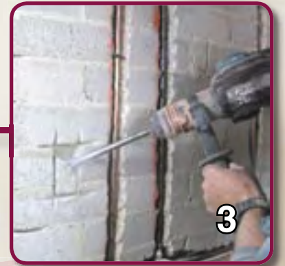
3. Chisel/hammer out brickwork to create wallbox cavity.
