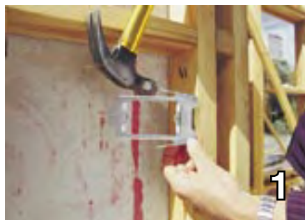
Installation of 155NAR Nail Bracket
