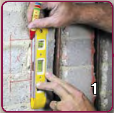
1. Mark out and drill wallbox position.
