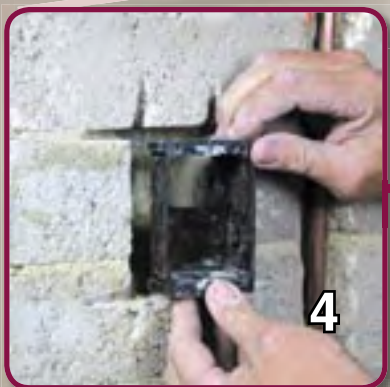
4. Insert wallbox and check wall recess has sufficient width and depth.
