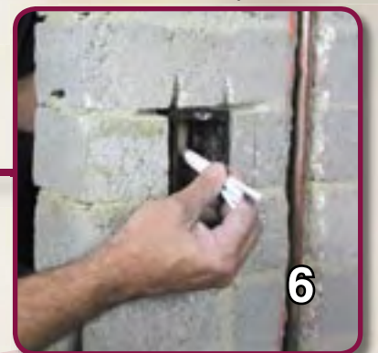
6. Run cable and insert through wall box.
