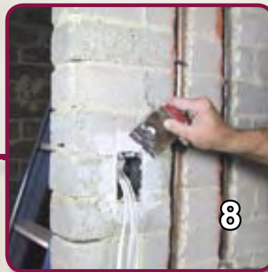
8. Finally, reinsert wallbox and apply wall filler
