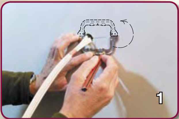
1. Mark out position for mounting 154 Mounting Clip. TIP: Turn bracket around and mark opposite side as guidance for a precise cutout.
