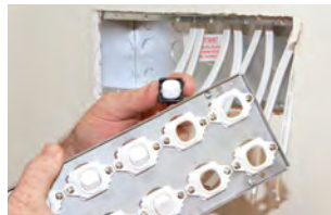
Step 5. Insert switch mechanisms (supplied separately) into grid plate.
