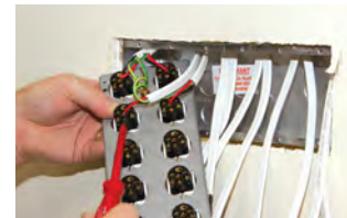
Step 6. Connect cables to switch mechanisms. Back off adjustment screws "Y" in grid plate.
