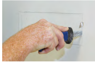
Step 2. Cut-out wall box position.
