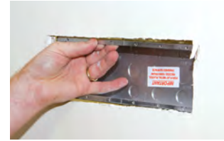
Step 3. Knock out appropriate cable entry points (ensure sharp edges are removed). Insert wall box.
