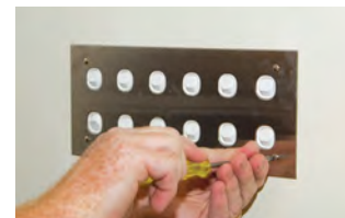
Step 9. Place metal fascia (cover plate) over mechanisms and secure with screws 'X' to grid plate.
