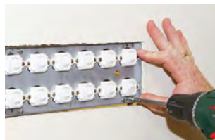
Step 8. Adjust screws 'Y' & 'Z' in and out until all shoulders on moulded mechanism clips align with finished wall face.
