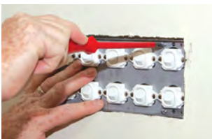
Step 7. Insert fixing screws 'Z' through grid plate and engage into wall box mounting holes. Place a straight edge on finished wall face across switch assemblies.
